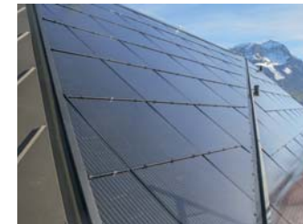
Flush fitted solar panels and roof ridge gutter
