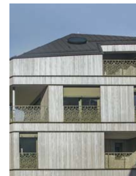
Facade with laser cut hand rail, wood surface
