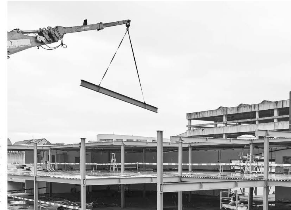
Abb. 4.09: Dismantling of the steel structure of an existing commercial hall in Basel. After dismantling, the components were processed and reused.
