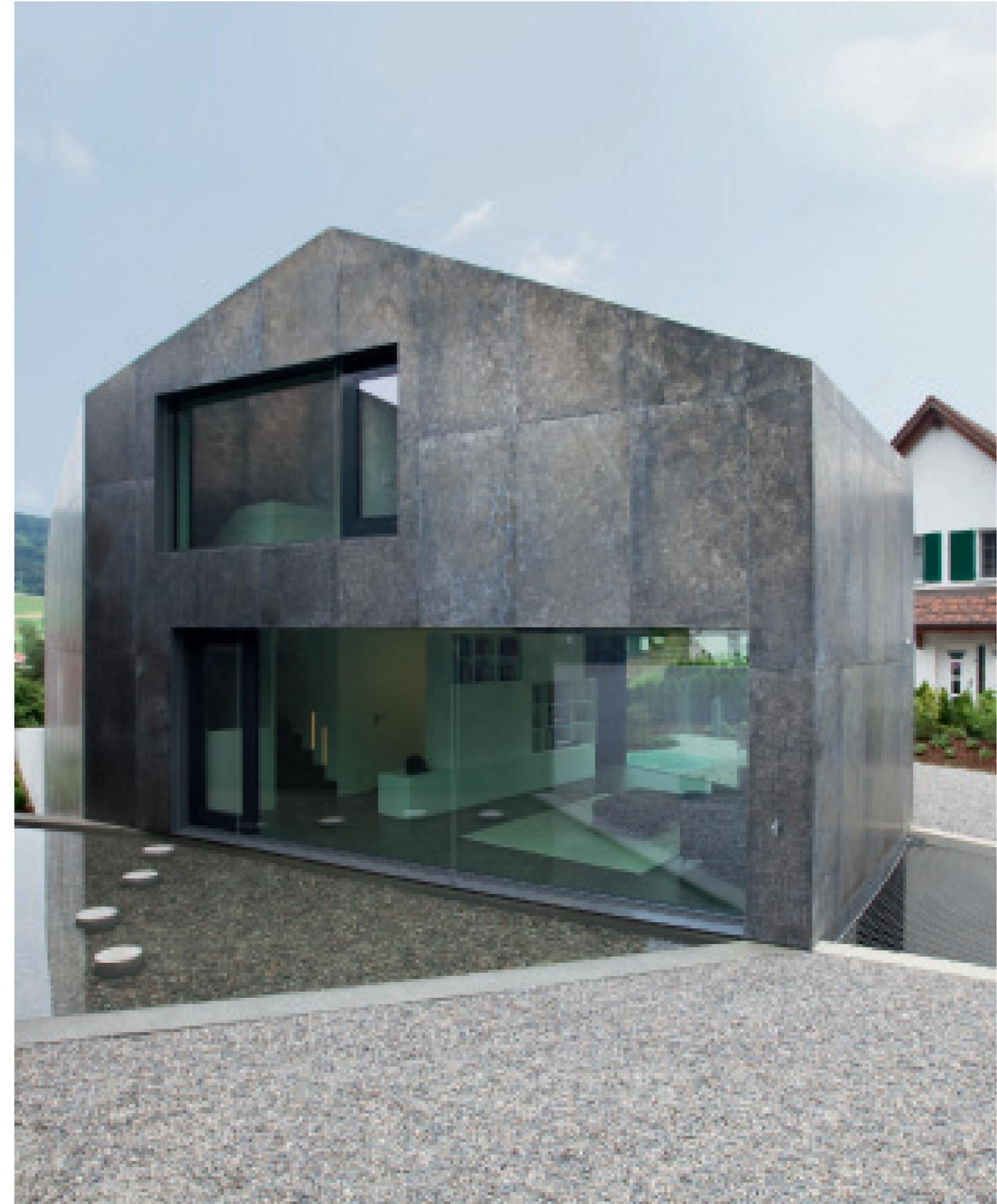
The architects fabricated a galvanized sheet with a unique and vital expression which was deployed for a first time on the façade and in the roof area.
